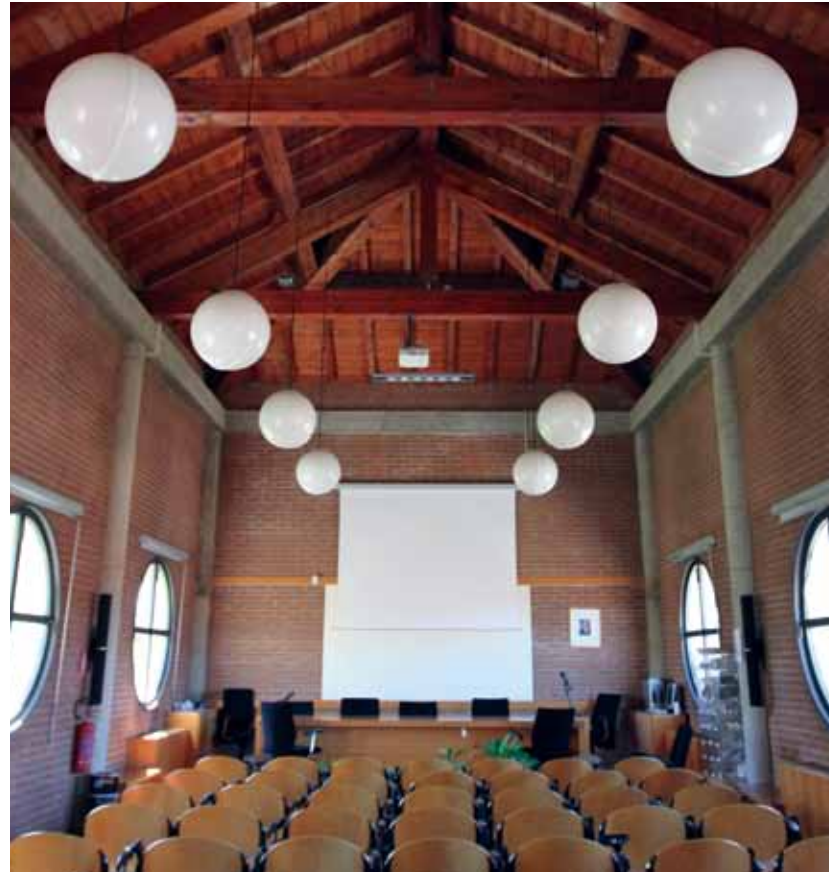
This conference room at CEM Ambiente SpA headquarters in Cavenago Brianza, Italy, is one of the many places within the revitalized landfill site powered by the five methane-gas fueled Capstone C65 microturbines.
